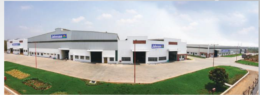
Johnson lifts factory complex in Sengadu, Chennai
