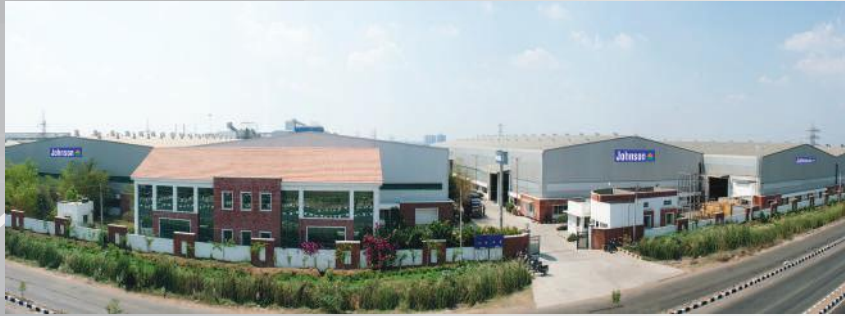
Johnson escalator factory complex in Oragadam, Chennai
