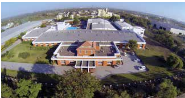
Johnson lifts factory, Nagpur
